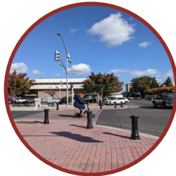
Curb Extensions Built with ADA Retrofits
